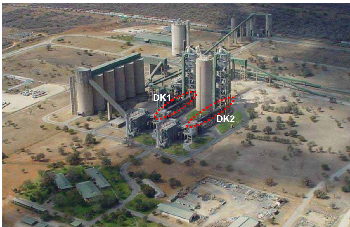
Figure 1-3: Aerial photograph of the future PPC Dwaalboom Manufacturing Plant, once construction has been completed; the positions of each kiln are indicated in red
