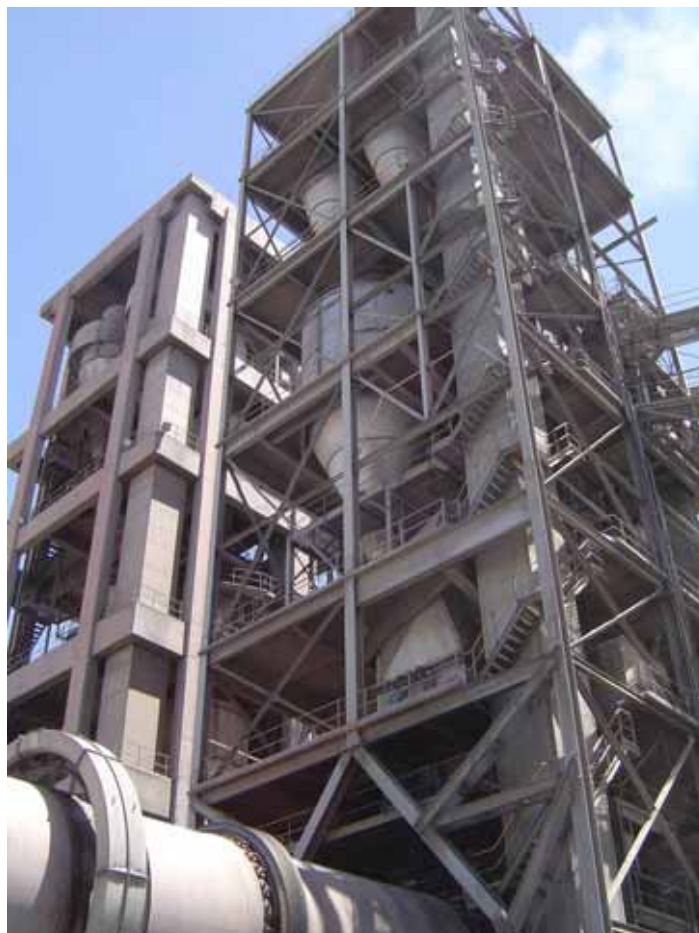
Figure 1-7: Photograph of a preheater at De Hoek.
