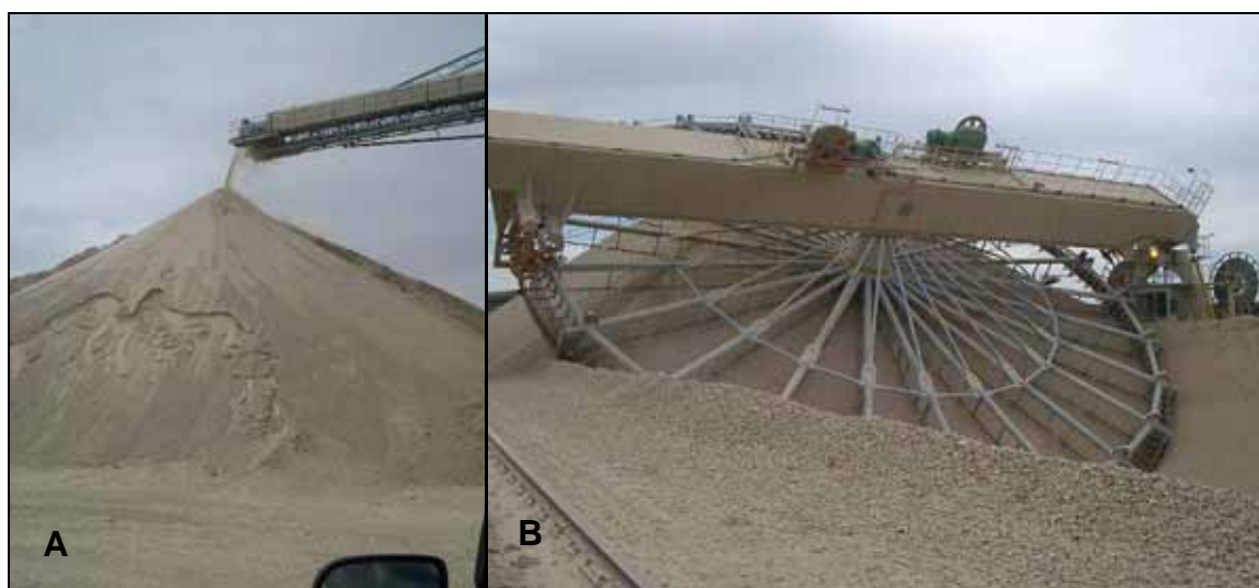
Figure 2-4: Photographs of the stockpiling of limestone at Dwaalboom (A), and the circular reclaimer (B)
