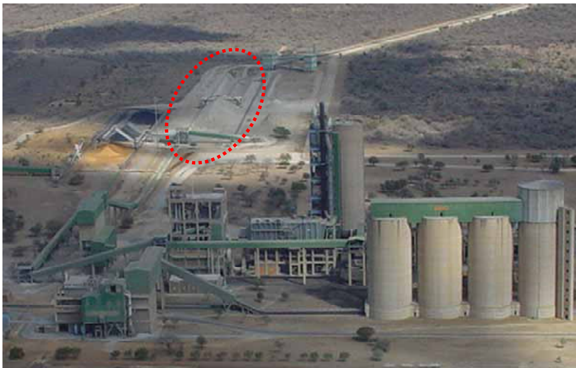
Figure 2-3: Aerial photograph of the limestone stockpiles at Dwaalboom, indicated in red. At the quarry, the limestone is crushed to particles approximately 25mm in size and stored on stockpiles, where the material is homogenised prior to milling.
