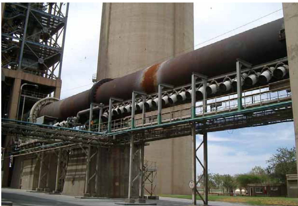
Figure 2-5: Photograph of the existing kiln at Dwaalboom; the raw meal silo is visible in the background
