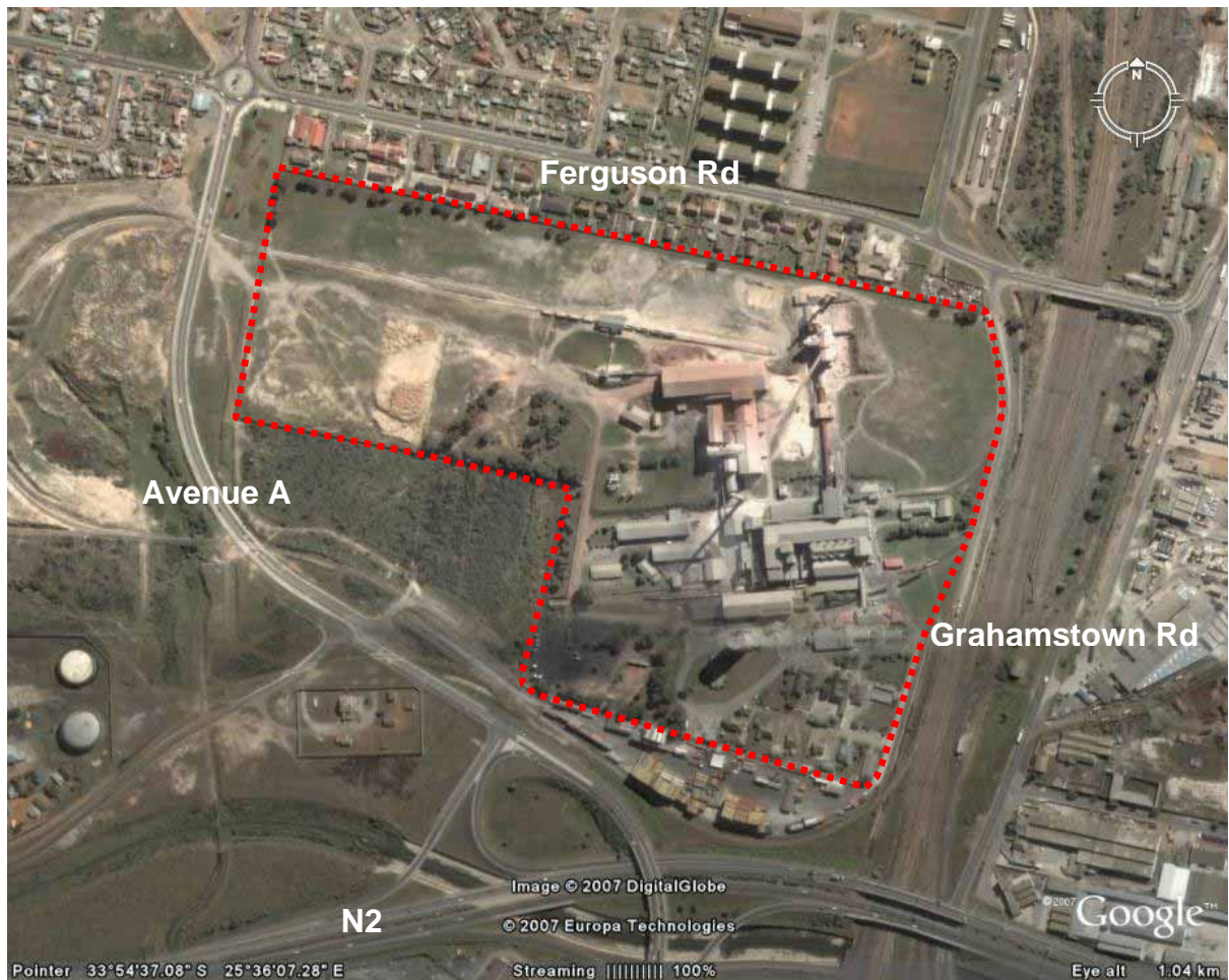
Figure 1-2: Google Image of the PPC Port Elizabeth Manufacturing Plant, showing adjacent roads.
