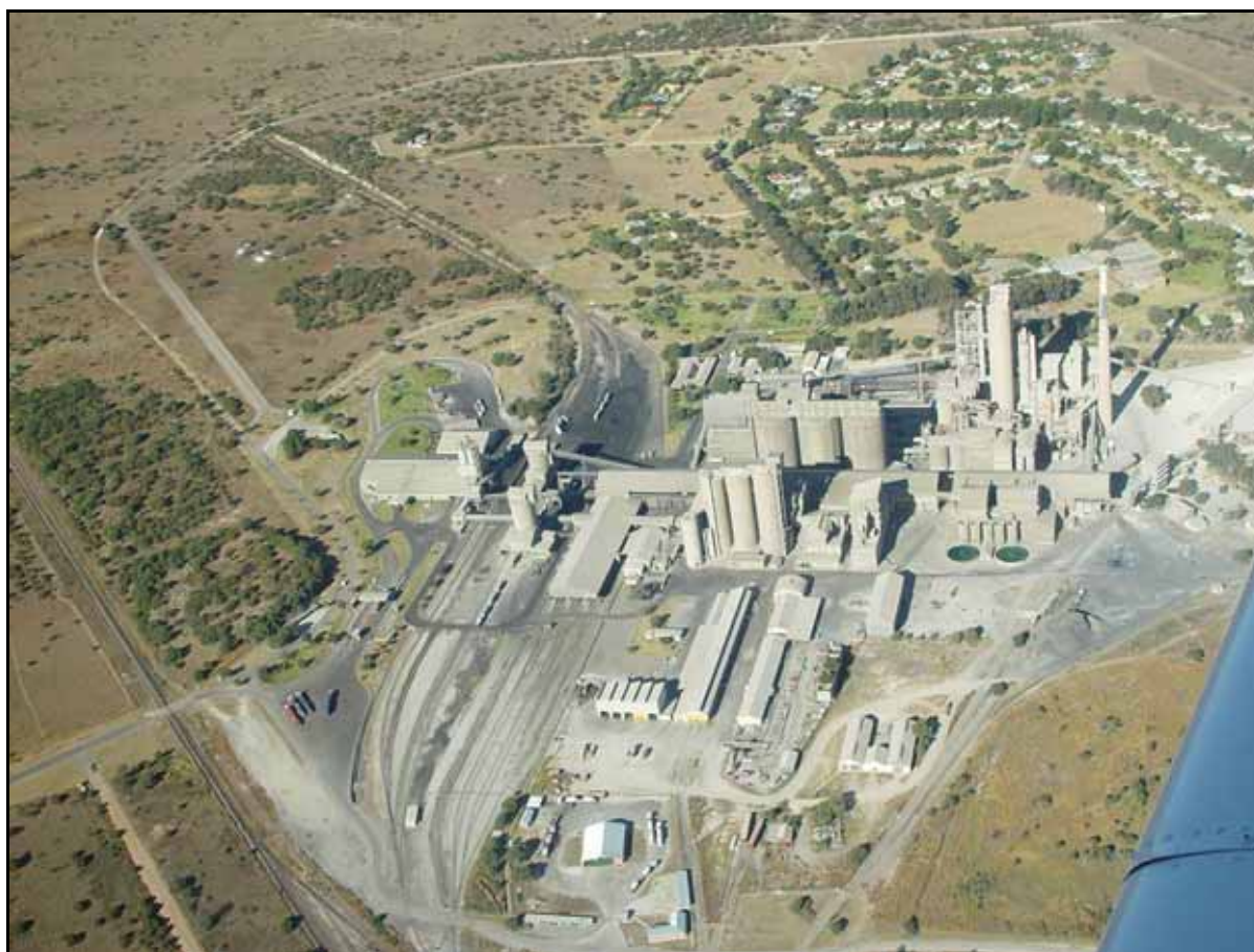
Figure 1-2: Aerial photograph of the PPC Slurry Manufacturing Plant
