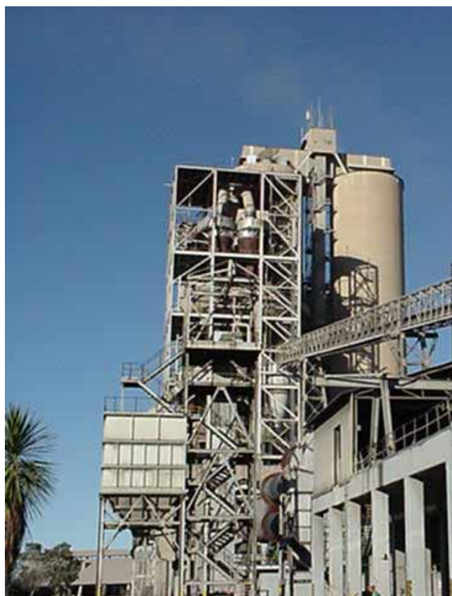
Figure 2-7: Photograph of the preheater of Kiln 8 at Slurry. The raw meal silo is pictured to the right of the preheater.
