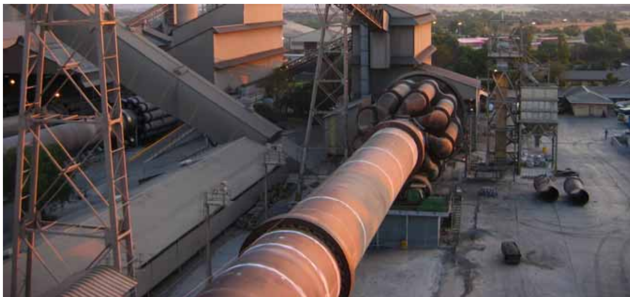
Figure 2-8: Photograph of Kiln 8, showing the planetary clinker cooler at the front of the kiln. Kiln 7 is visible in the left of the photograph.
