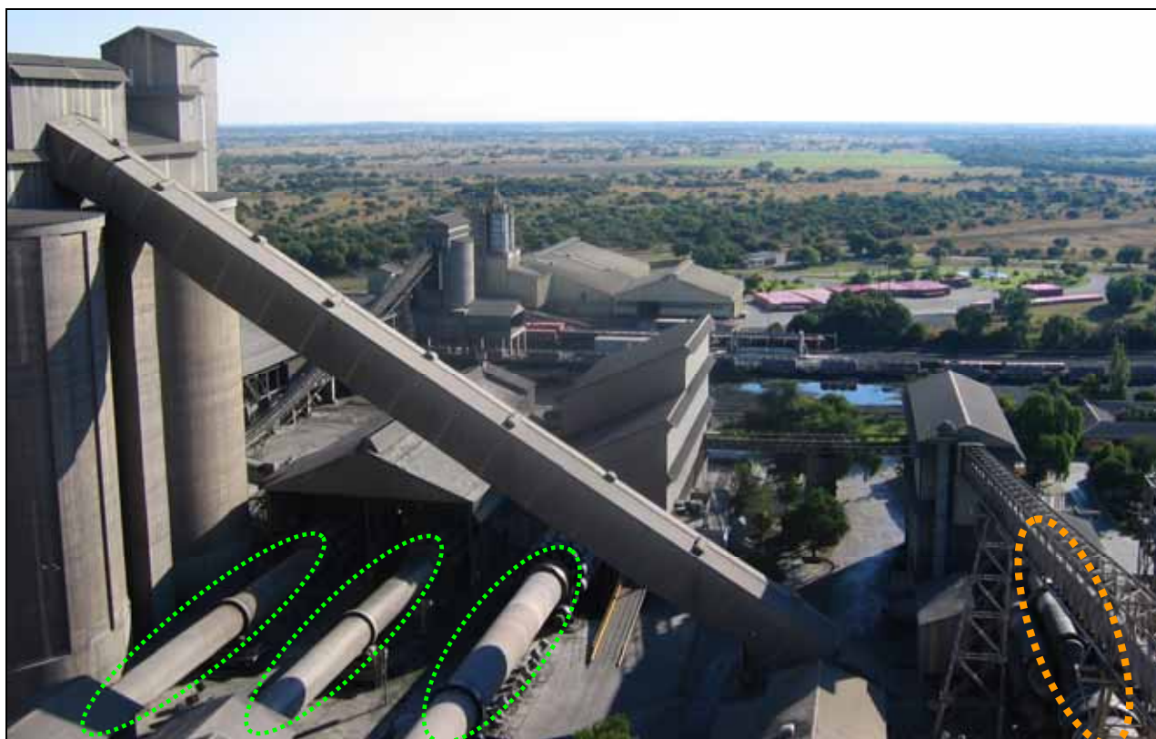
Figure 2-6: Photograph of the Slurry factory showing the four kilns, from left to right: SK5, SK6, SK7 (as indicated in green) and SK8 (indicated in orange).
